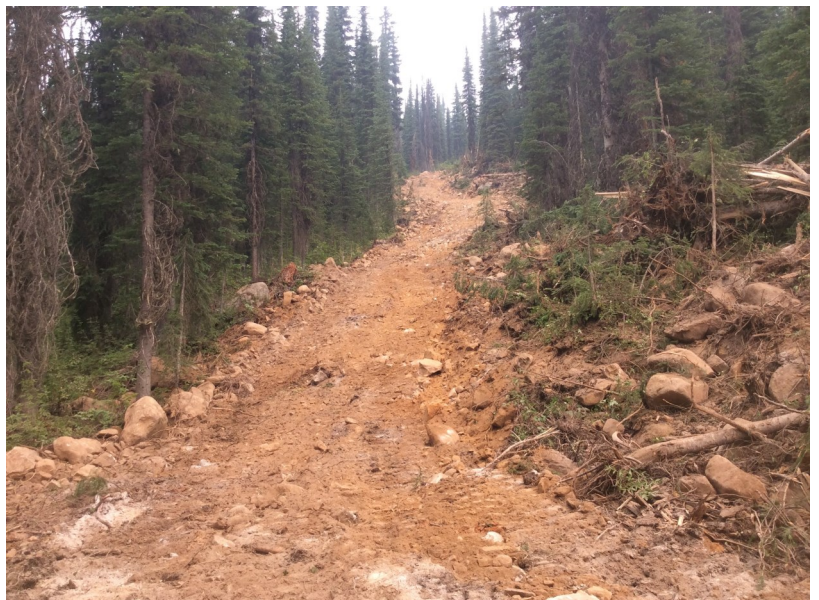
Control line located on the east flank of Octopus Creek Wildfire (July 31, 2021)
